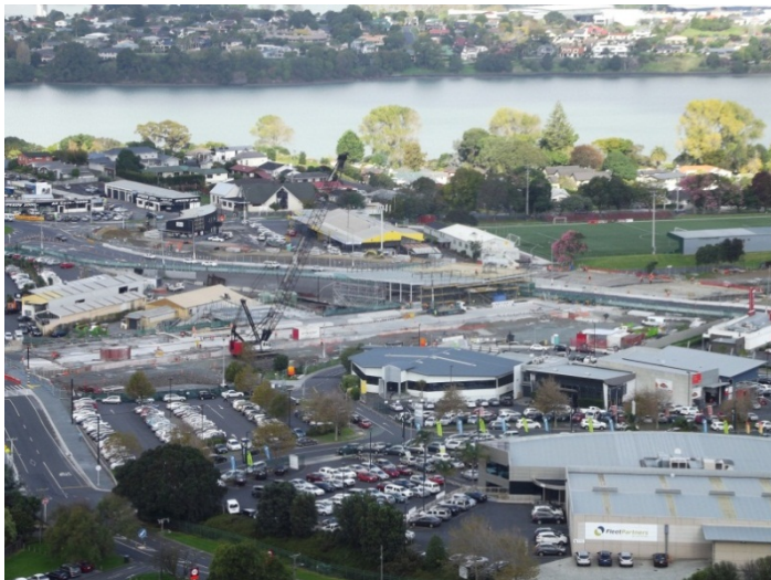
Fig 2: Construction site progress - view from Mt Wellington
