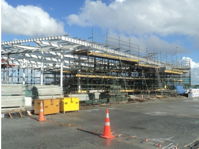
Fig 1: Panmure Station steel superstructure erected
