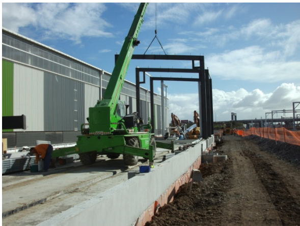
Fig 5: Erection of structural steelwork for the train wash building
