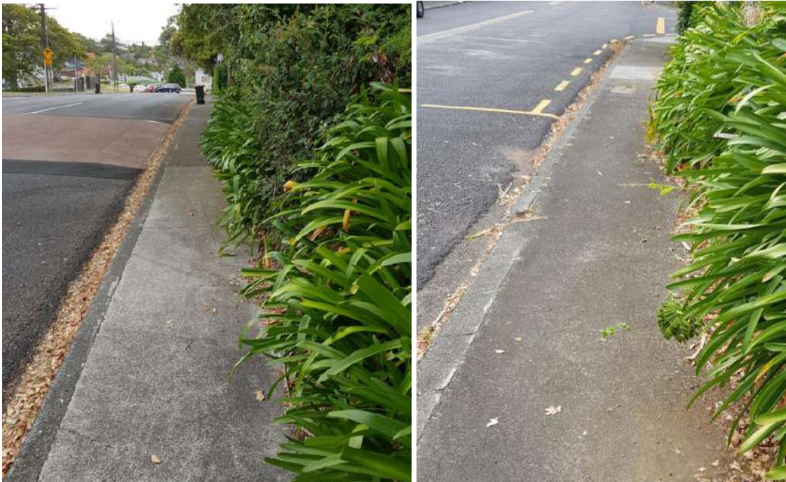
Figure 8: Overgrown vegetation reducing the usable width of the footpath.
