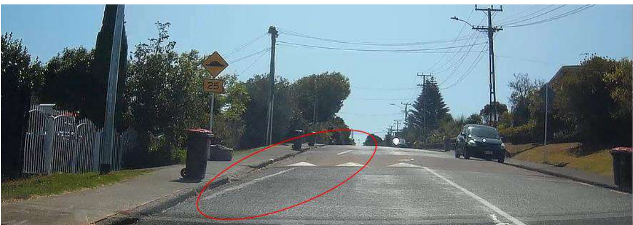
Figure 14: Redundant centreline, RRPMS still visible on site and redundant table still visible on site.
