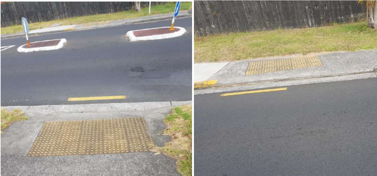
Figure 15: Refuge Island and the higher kerb lip
