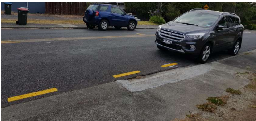
Figure 24: View to the right from the access near the bus stop on the westbound direction near school indicating that parking already limits the sight distance to the right.
