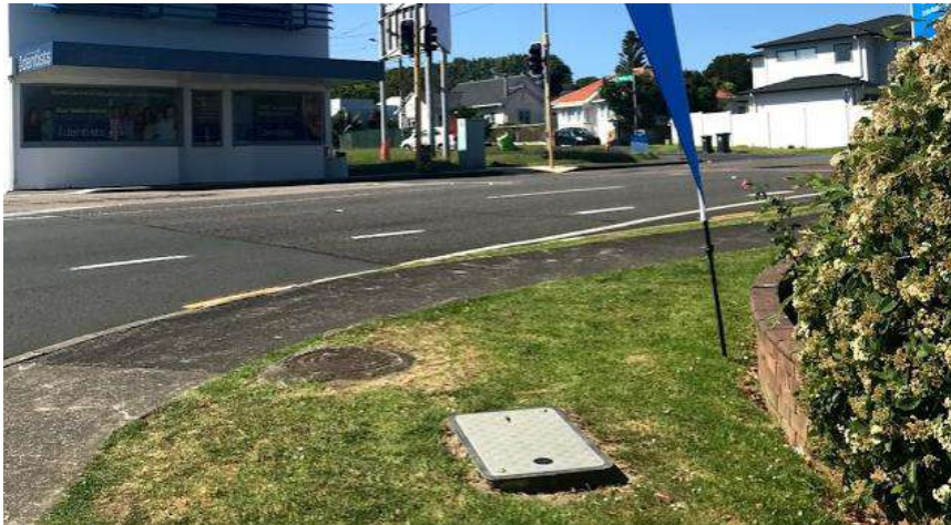
Figure 19: Limited sight distance for pedestrians crossing Littlejohn Street
