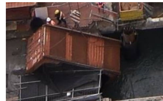
Container has gone over the edge of the wharf
