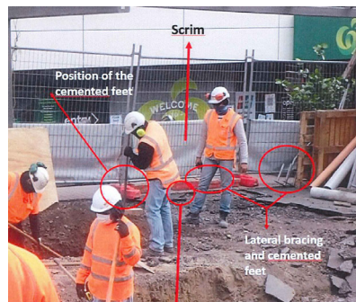
Fencing being dismantled and moved
