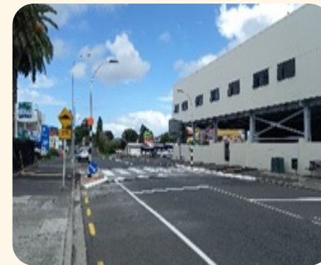
Completed raised zebra crossing at Kolmar Road, Papatoetoe
