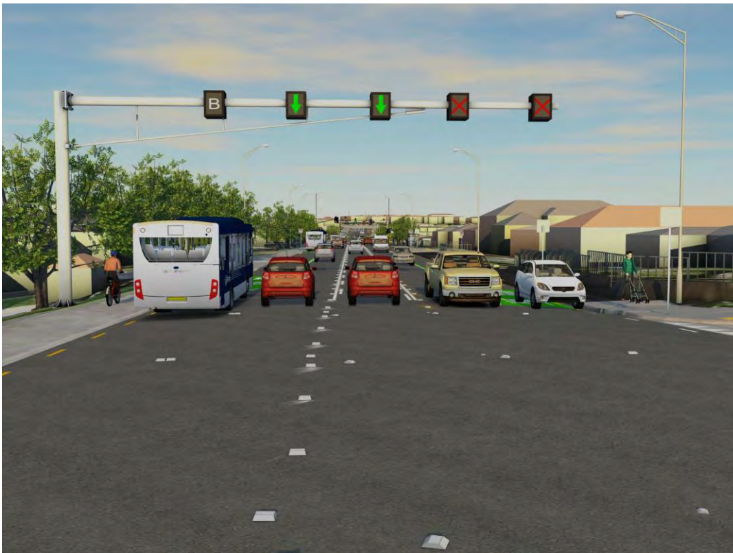
Model impression of dynamic lanes on Maioro Street, view towards the West
