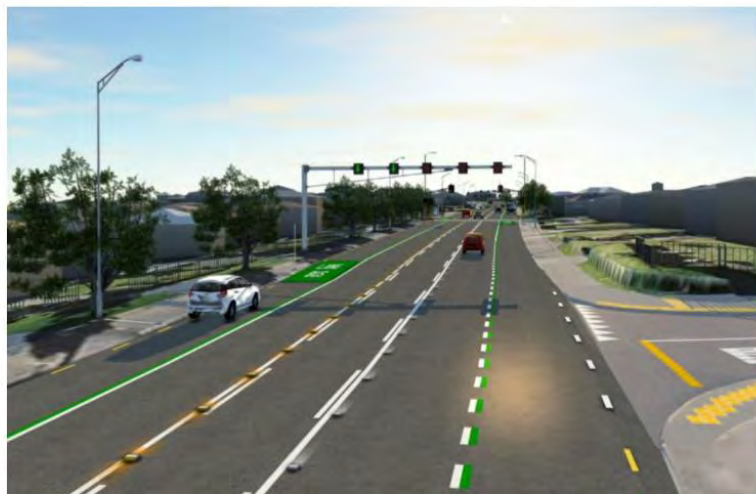
1. Dynamic Lanes on Maioro Street
