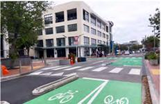
The intersection of Market Place and Customs Street West has been raised, with a pedestrian crossing on each intersection leg, providing three safe crossing points.
