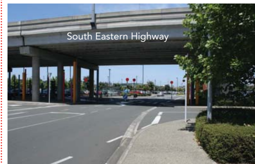
Above: Sylvia Park bus interchange before improvements
